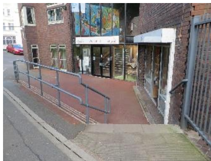
Rear door accessible by a few steps...
