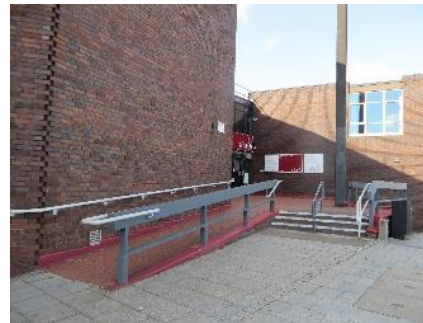
Slope or steps to access the front door on Moor Street Queensway
