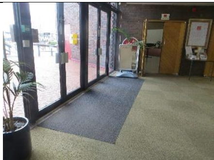
Floor at main door into church
