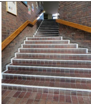
Floor and brick steps from rear door access
